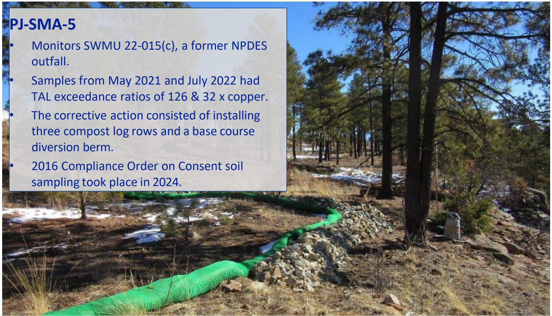
Rock check dam J00506010024, compost log J00506010028, and sampler at PJ-SMA-5.
