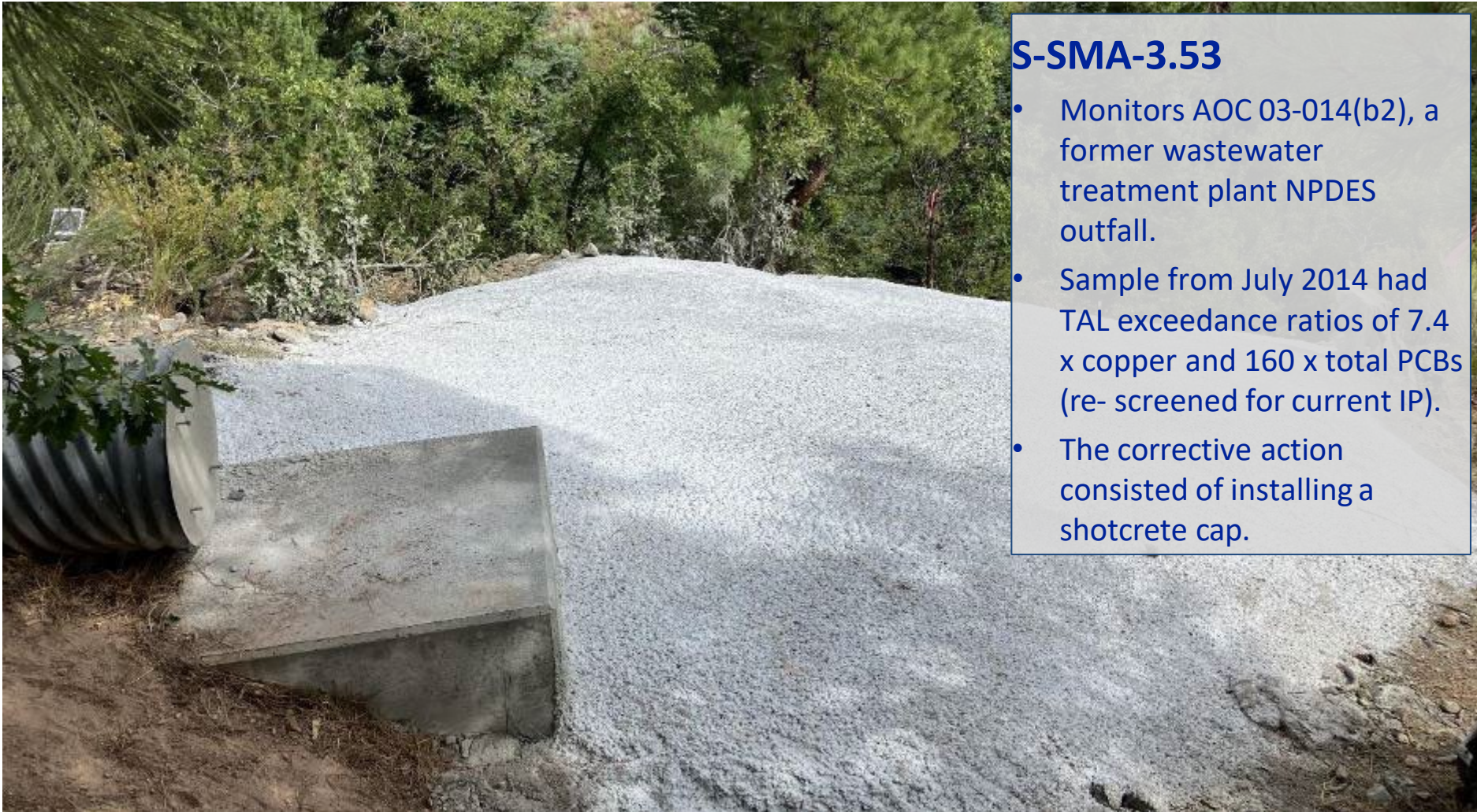
Shotcrete cap S005B08030008 at S-SMA-3.53.
