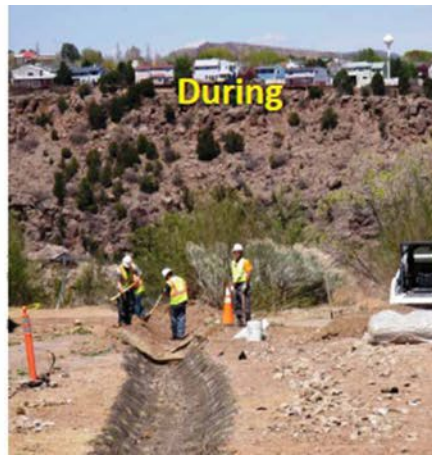
Installation of storm water controls as a corrective action at P-SMA-2.2 in 2011
