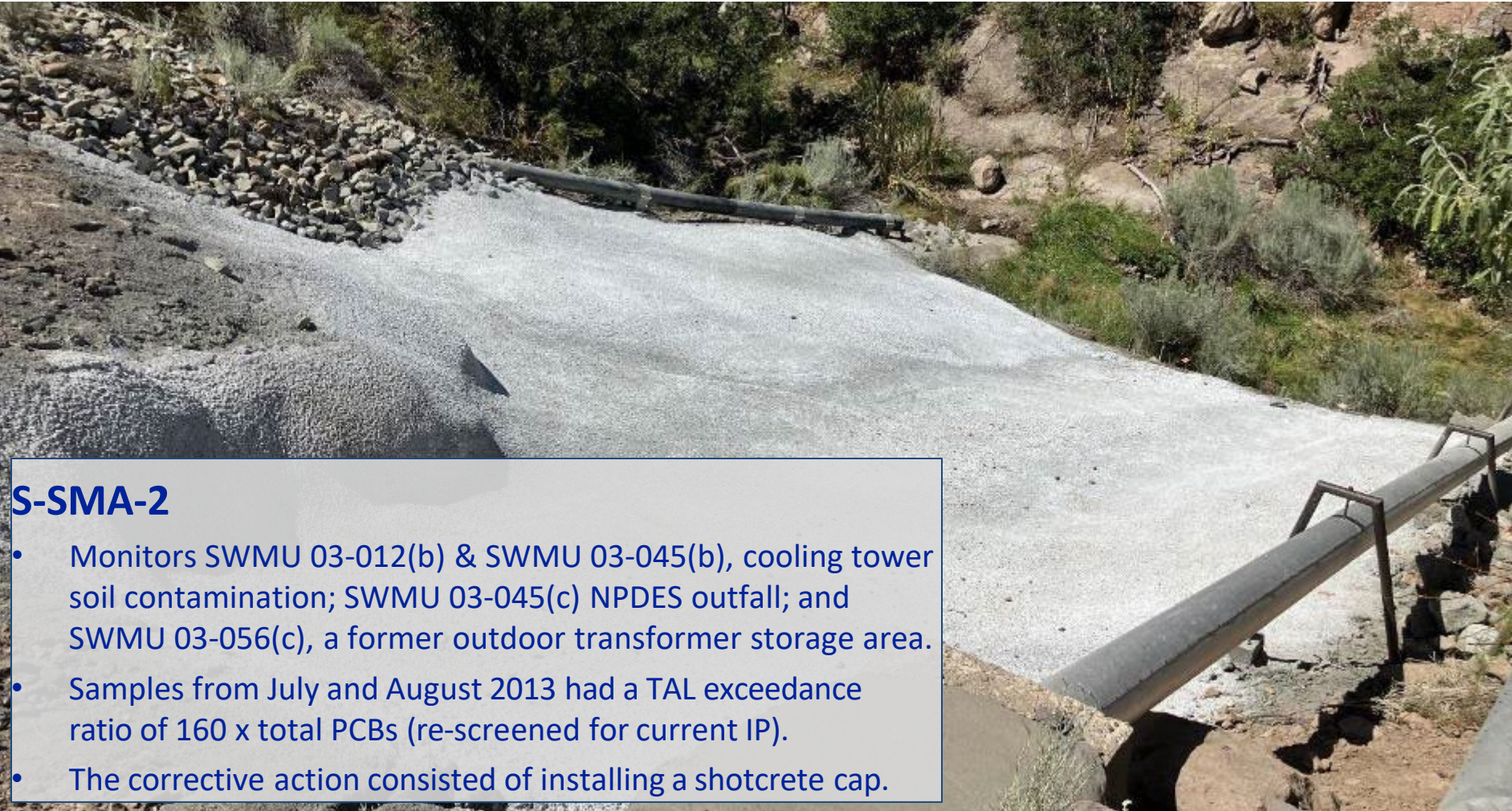
Shotcrete cap S00308060028 at S-SMA-2.
