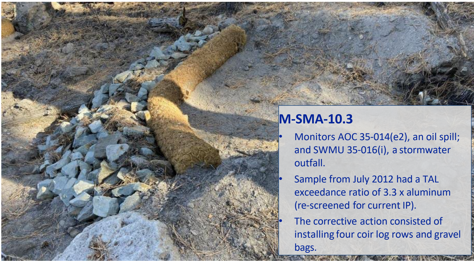
Rock check dam M01306010017 and coir log M01306010023 at M-SMA-10.3.
